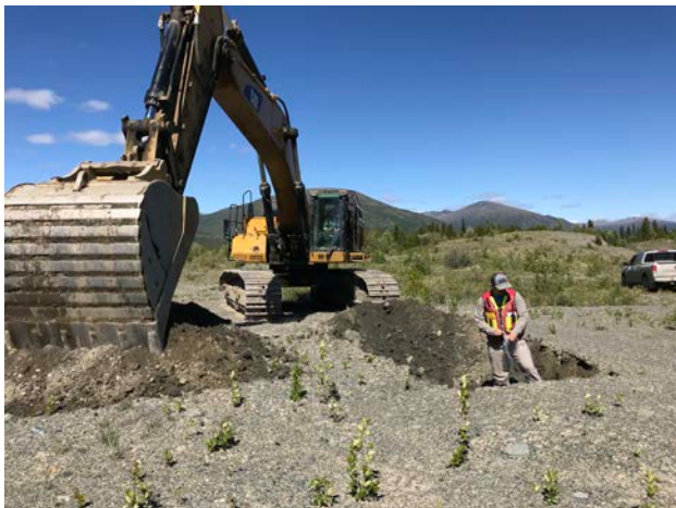
Test pits program on proposed power canal.
