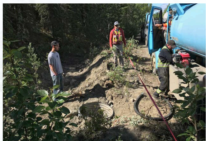
Performing seepage testing in the power canal during the feasibility study.
