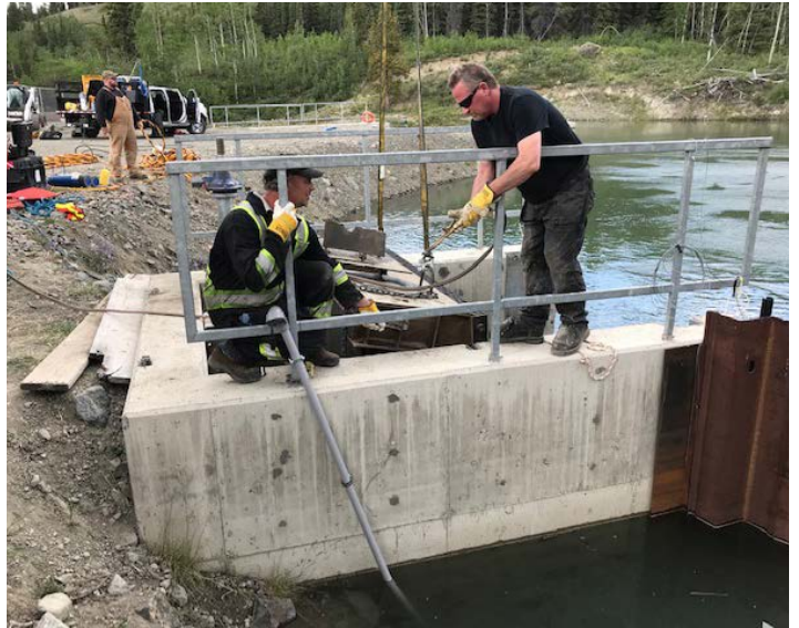
Maintenance work at the existing headpond and intake structure.
