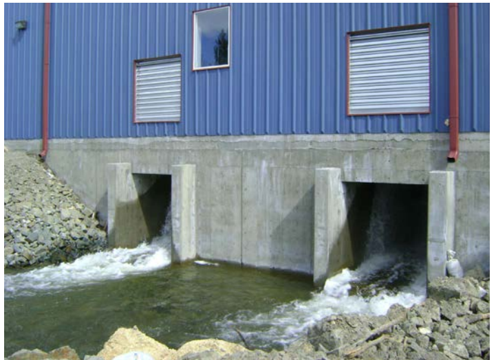
Tailrace at existing powerhouse.
