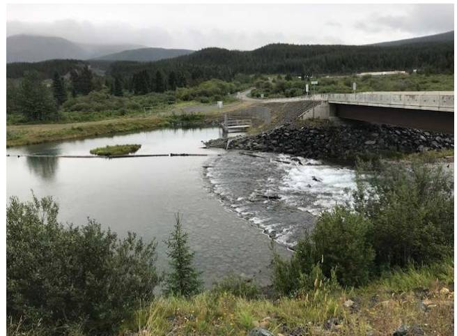
Rockfill weir at Surprise Lake
