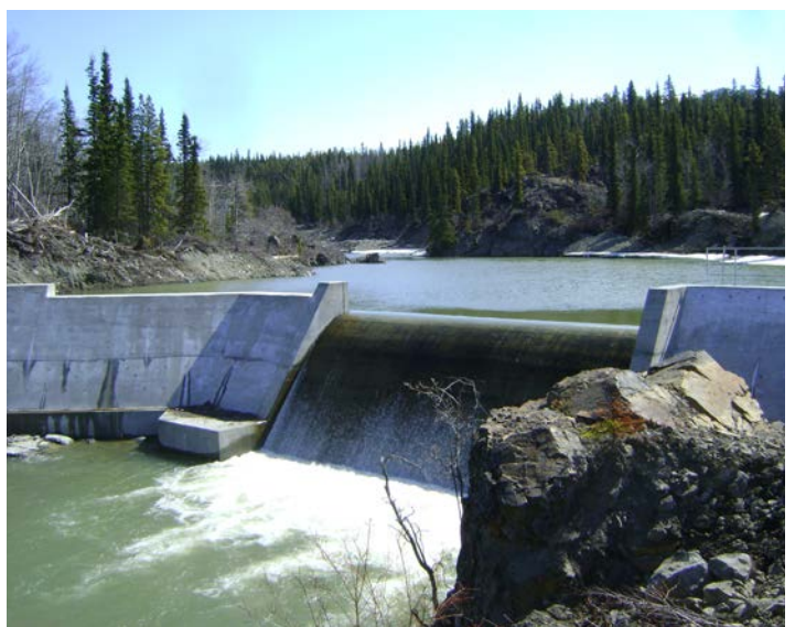
Existing concrete dam.
