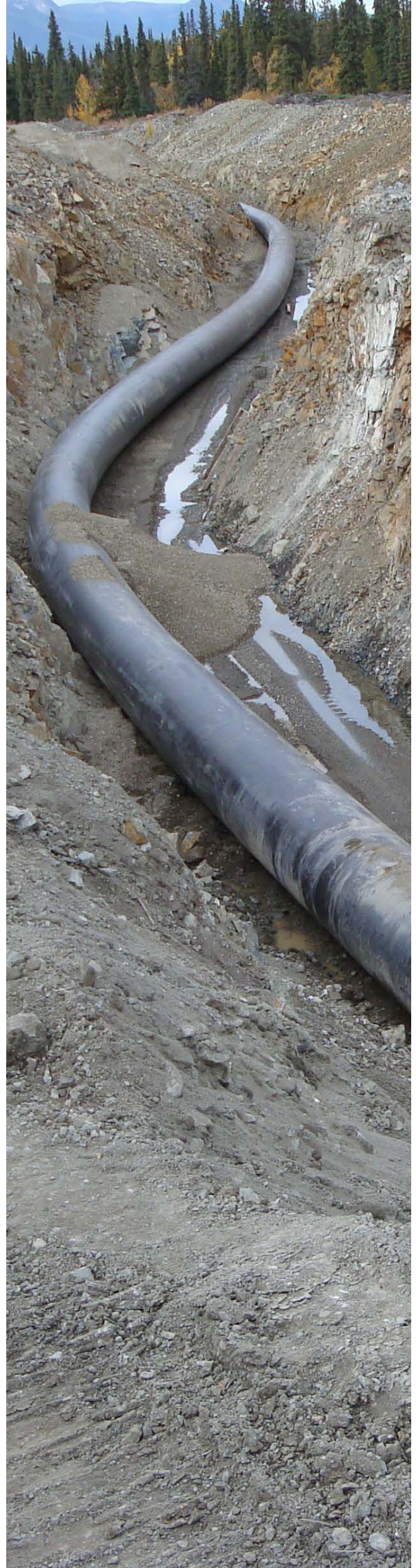
Construction of existing penstock pipe.
