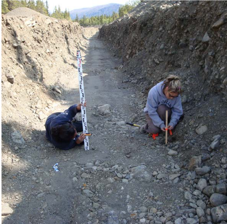
Surveying of existing penstock.
